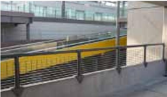
Additionally, at London Gatwick Airport, BSG has been contracted to supply gratings and tubular fittings to construct parapet barriers within a new multi-storey car park. All the items are powder coated and this bespoke product is a first for BSG, utilising this size of grating in a vertical rather than horizontal plane.
